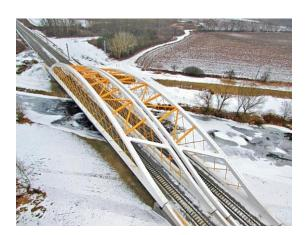
The reconstruction consisted in the removal of a technically unsuitable bridge at km 80,930 of the railway line and provision of the requested railway line speed of 160 km/hour. The original three consecutive structures were replaced with a bridge with a single opening, as requested by the Morava River Basin Agency.
