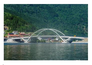
Loftesnesbrui is a 194-meter-long steel bridge, situated in the town of Sogndal by the Sognefjord. The bridge has a network tied arc in the main span, and the middle of the arc is 15 meters high, from top to bottom. The new Loftesnesbrui bridge was built because the old bridge over the Loftesnes sound was very narrow, and it was starting to show signs of wear and tear. The bridge from 1958 had almost no space for pedestrians.
