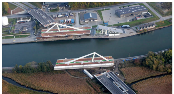
Areal view of the bridge and the administration building. The foundations are placed in a position so that the open bridge lies within the shoreline of the canal, giving maximum width of the canal to ship traffic thus eliminating risk of collision.
