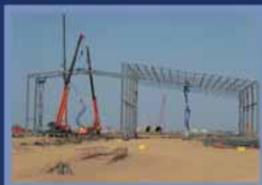
Medupi Power Station
