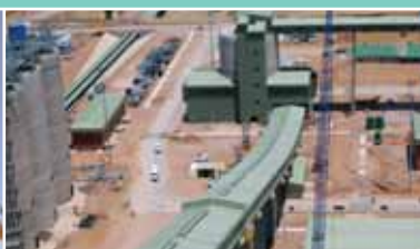
Medupi Power Station – Coal and Ash Terrace
