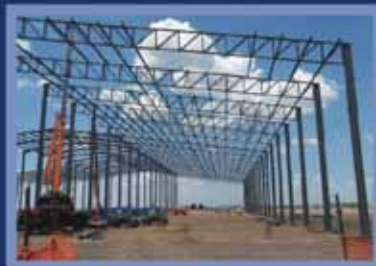
Medupi Power Station
