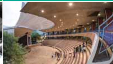
University of Pretoria Amfi Roof Structure
