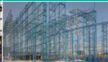
New Ferrochrome Furnaces Factory
