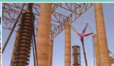
Medupi Power Station – Air Cooled Condenser
