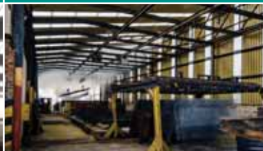
ARMCO Galvanizers Boksburg - Refurbished Roof over Process Tanks
