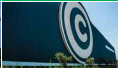
Cell C Warehouse, Midrand
