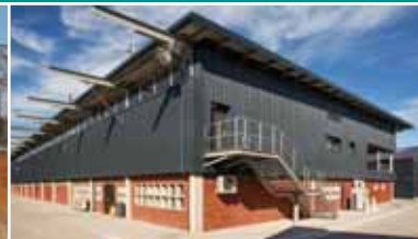
Ndabeni Electrical Depot
