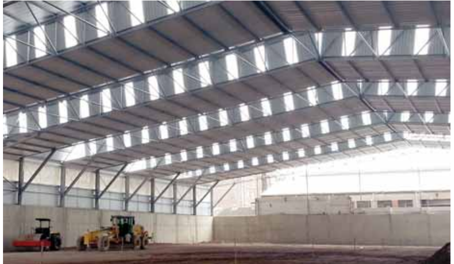
Photographs: Cousins Steel International (Pty) Ltd
