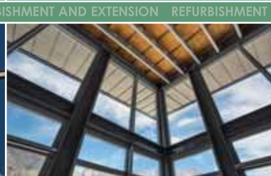
Roeland Park Office Block Development
