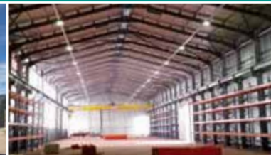
Warehouse Upgrade Kumba
