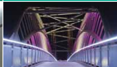
Davenport Road Bridge
