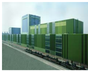
Hot Dip Galvanizing Line Dortmund
