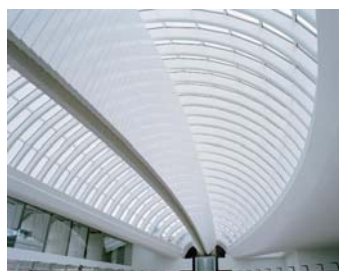
Roof of the University Zurich
