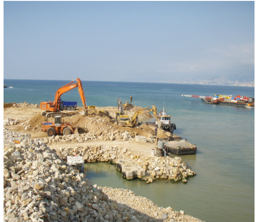
RECLAMATION WITH SPLITBARGE
