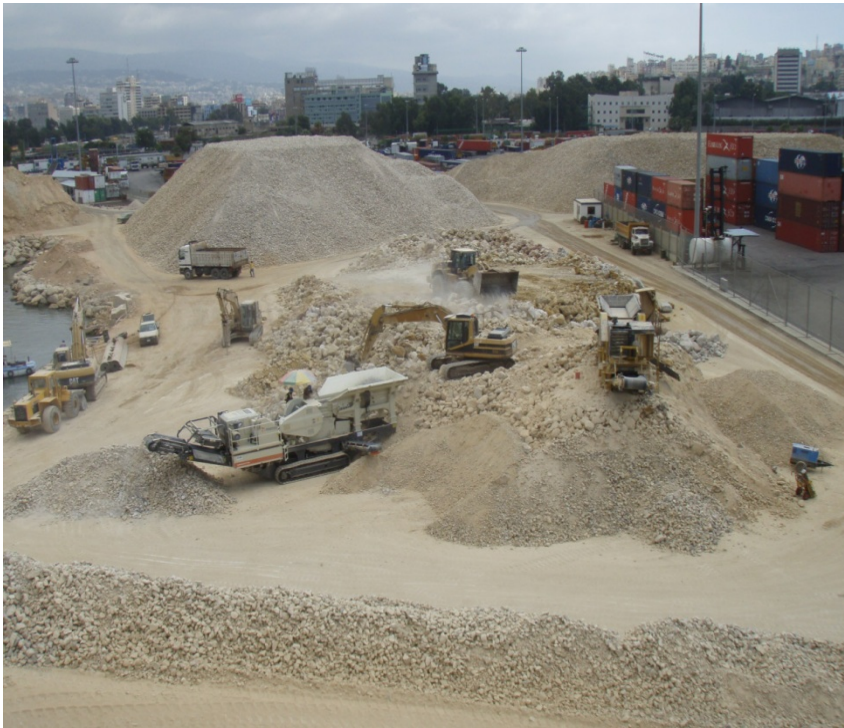
CRUSHING – FILL MATERIALS
